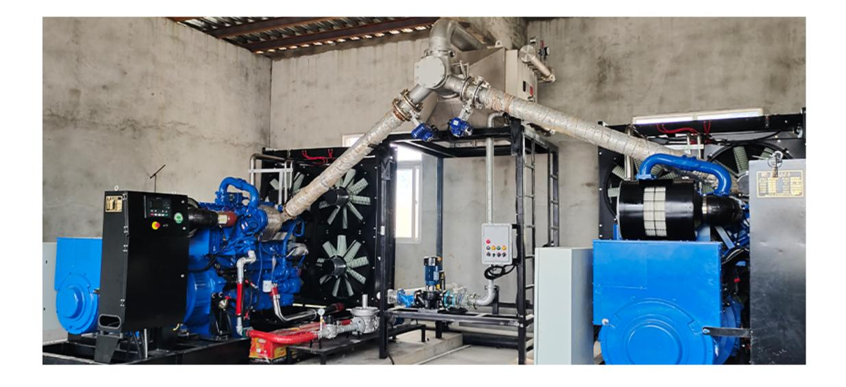
The plant is located in Chongqing, China, and adopts 2\* 320KW cogeneration generator sets. The isolated network operation of the unit provides continuous power supply for the pig farm for 24
