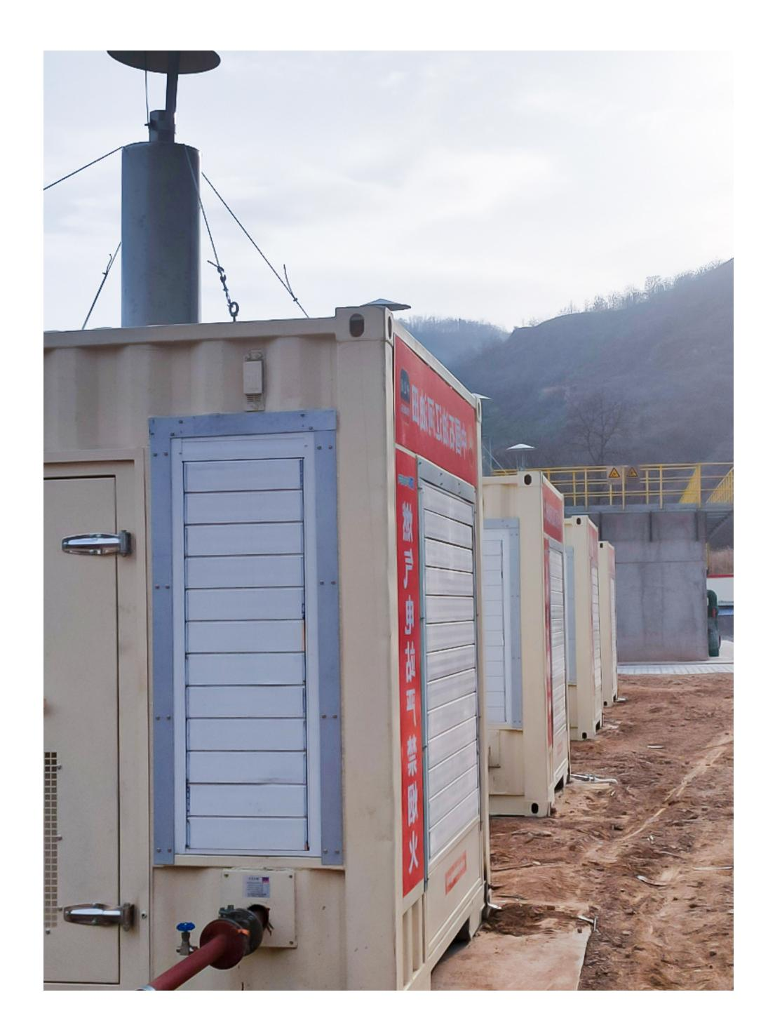
Located in Linfen city, Shanxi Province, CNPC Liaohe Oilfield's CBM power generation project uses 8\*250kW (total power 2MW) container-type gas generating units. The power generated by the units is integrated into the local oilfield grid to provide power for drilling and pumping units in the surrounding area.
